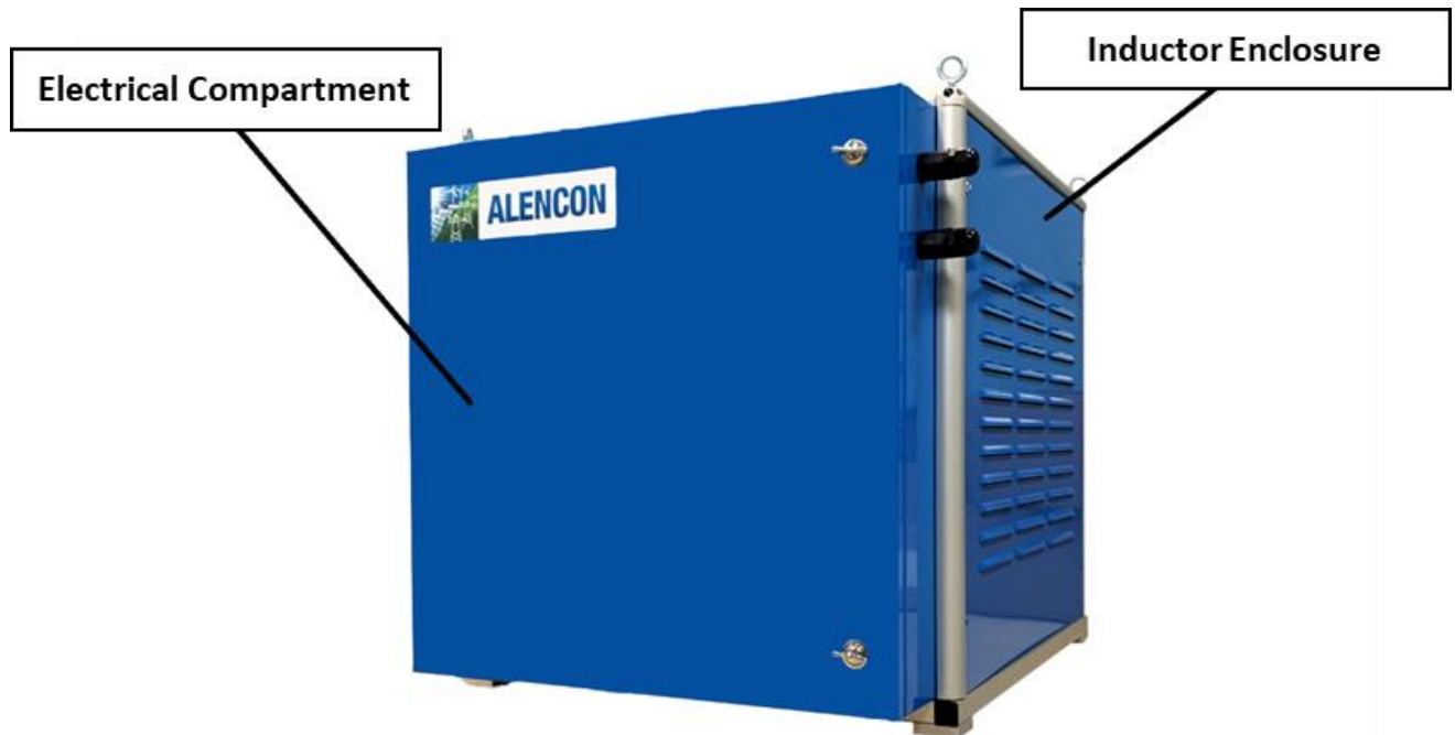
FIGURE 7: CUBE – TWO SECTIONS
