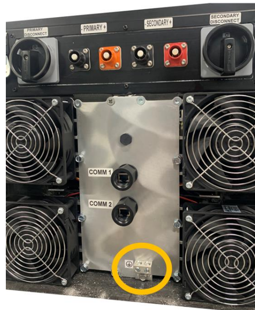
FIGURE 18: SPOT/BOSS UNIT GROUNDING
