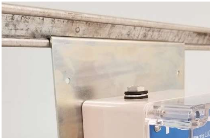
Figure 9: Hook shaped PODD mounting bracket on Unistrut® support
