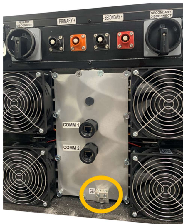
FIGURE 19: BOSS GROUND LUG LOCATION EXAMPLE (IN ORANGE)
