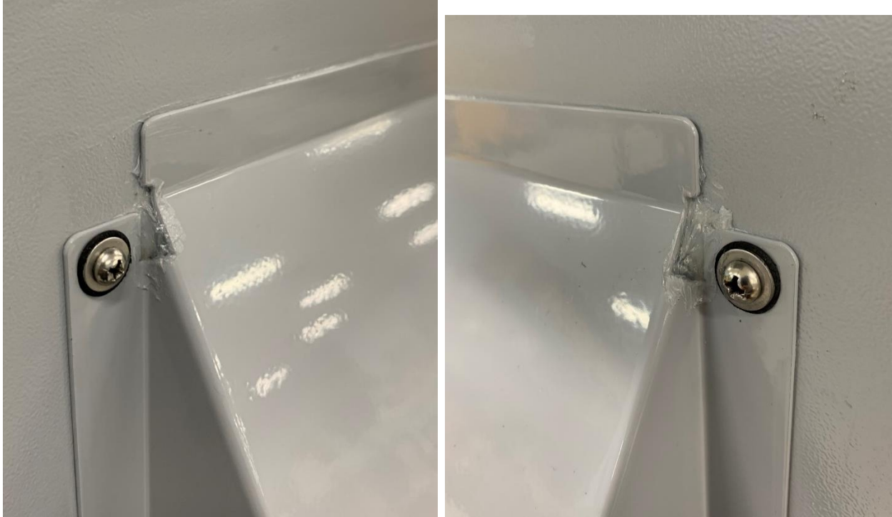
FIGURE 42: SILICONE CAULK SEAL ON DOOR HOODS
