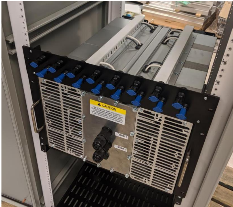
Figure 10: H4/MC4 Termination
