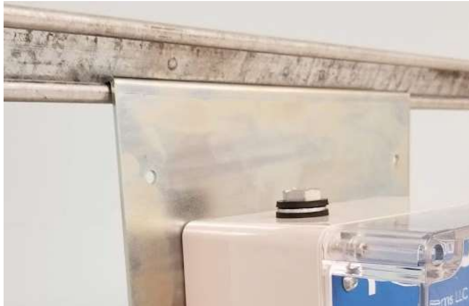
Figure 11: Hook shaped PODD mounting bracket on Unistrut® support
